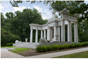
Thomas H. Swope Memorial Monument Restoration City of Kansas City, Missouri
