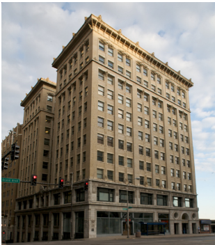
Scarritt Building and Scarritt Arcade Restoration / Rehabilitation Kansas City, Missouri
